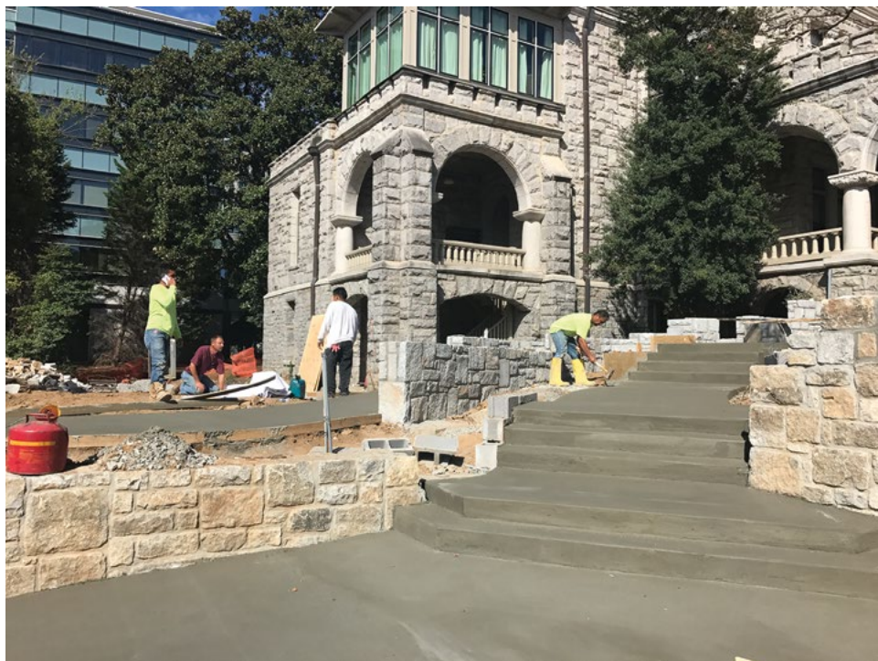
Rhodes Hall is undergoing a significant rehabilitation of the grounds to alleviate issues with drainage, erosion, grading and poor plantings. Pictured is a new hardscape being installed in the back to improve accessibility.
