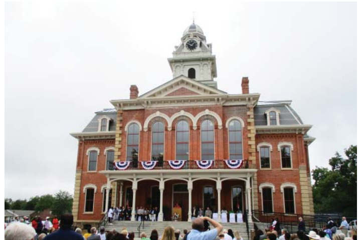
Hancock County Courthouse, Sparta
