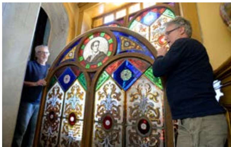
The Lord Byron window at Hay House in Macon was removed for repairs after it was damaged during a storm in July 2016.
