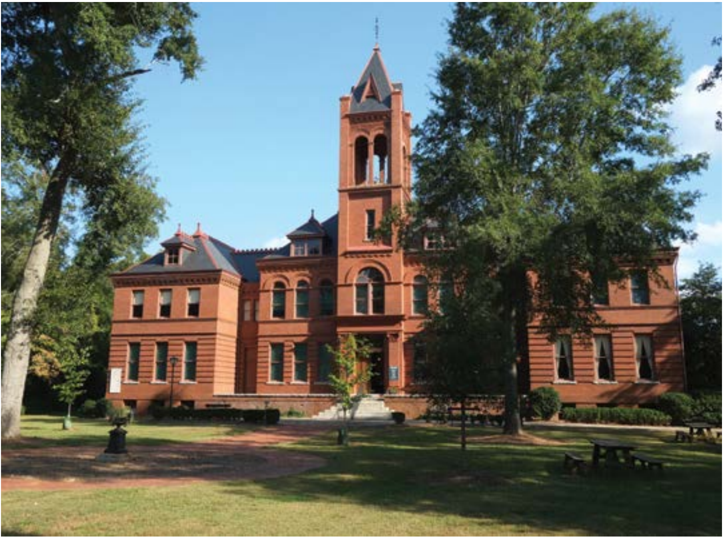
Since completion of a sustainable rehabilitation, the Madison-Morgan Cultural Center has seen a 35% decrease in their utility bills.
